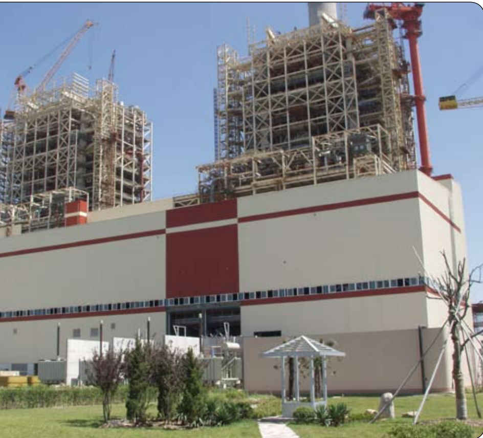
Wai GaoQiao coal power station near completion
